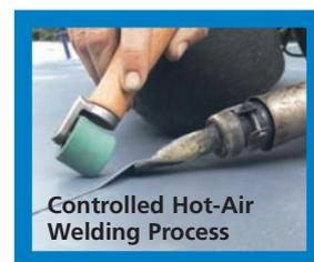
Controlled Hot-Air Welding Process
