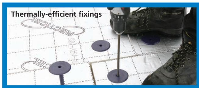
To counter this, we've developed a new fixing method for all Vanguard installations. The metal screw is placed inside a special thermally-efficient tube, that's counter-sunk within the body of the insulation.
